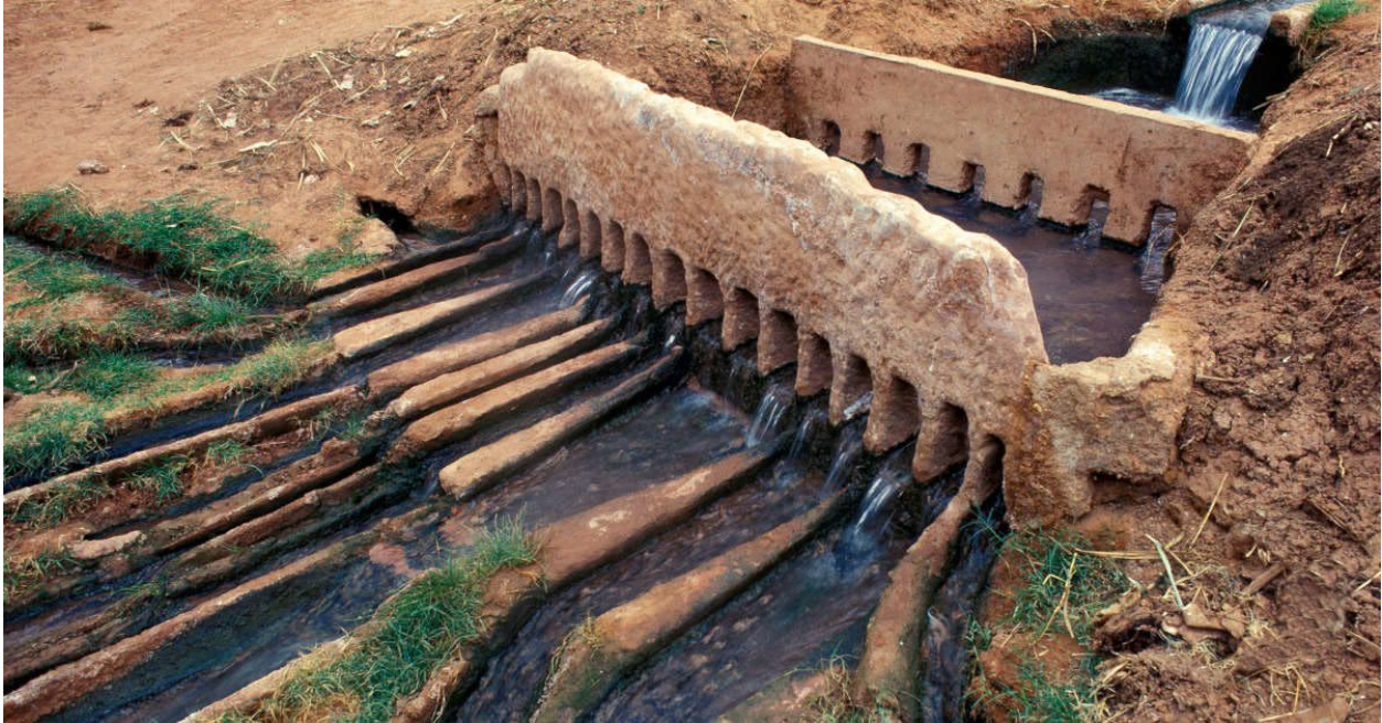
Water flowing through a distribution weir on a foggara, an irrigation system developed approximately 3000 BCE in the Near East region.
