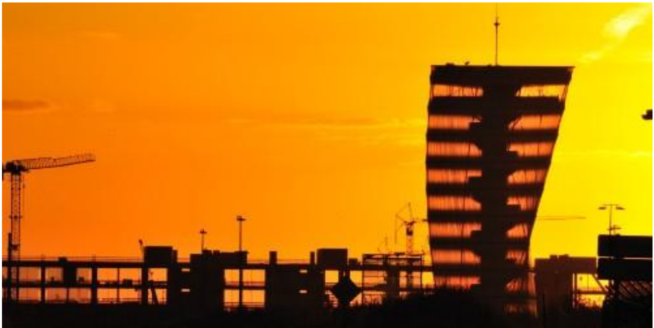
Infotower with 360° webcam system, BER Airport Construction Site, Kusus+Kusus Architekten
