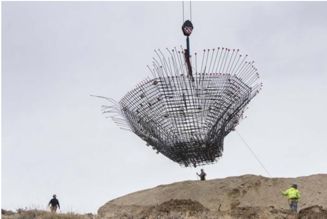
Construction of Structures of Landscape, Ensemble Studio
