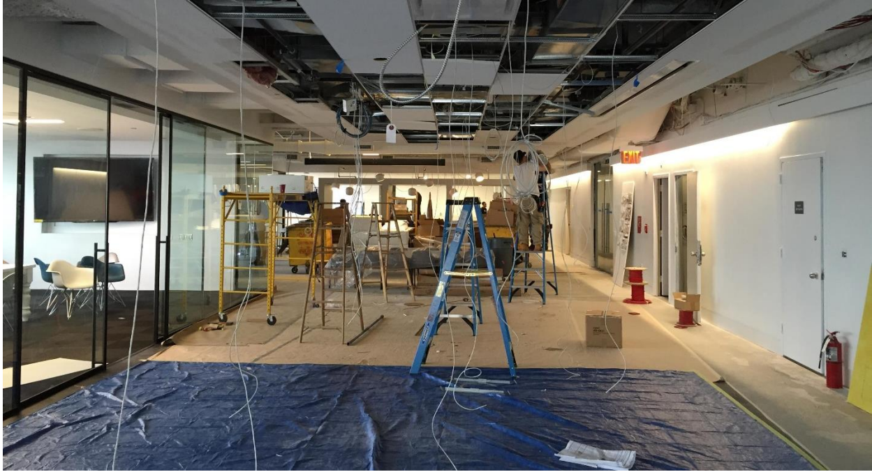
Office Fit-out Progress (Photo Najeeb Hameen)
