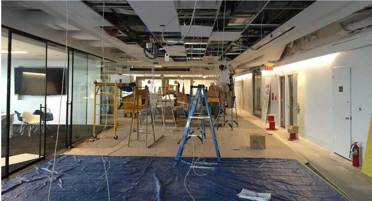
Office Fit-out Progress (Photo Najeeb Hameen)
