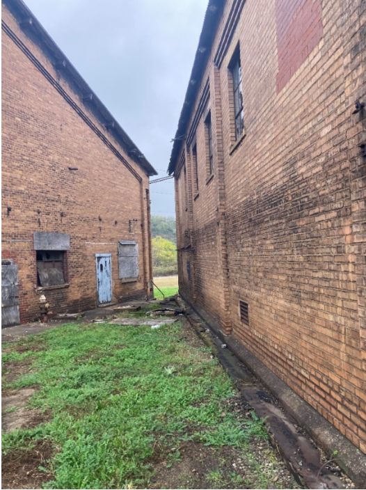
Figure 6.10: East wall of McKeesport Roundhouse (left) and adjacent building (right)
