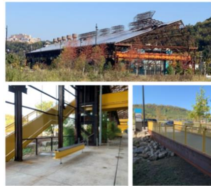
Fig 3.5 Steel Reused on Site (Image Source: Shah, 2022)
