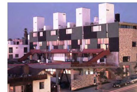
Left: Yokohama apartments by ON design (Photo: © koichi torimura) Top right: City in the Making, Rotterdam by Stealth.unlimited Bottom right: The Essex Apartments, San Diego by Ted Smith & Others
