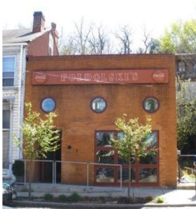
Figure 6 Front of building
