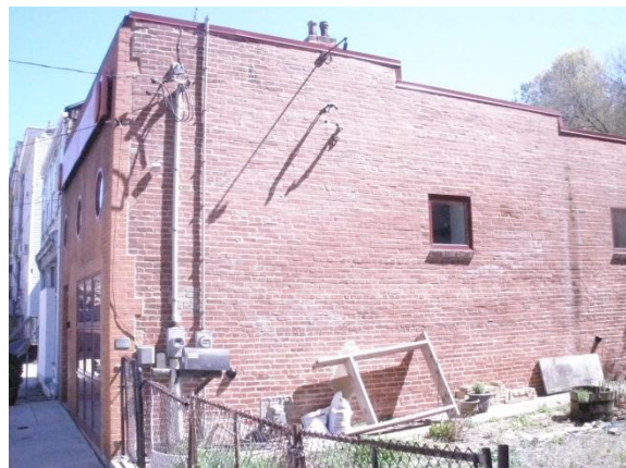
Figure 39 Windows on western Wall
