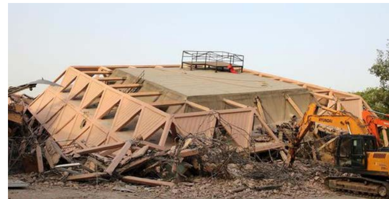
Demolition of the Hall of Nations by Raj Rewal, April 2017
