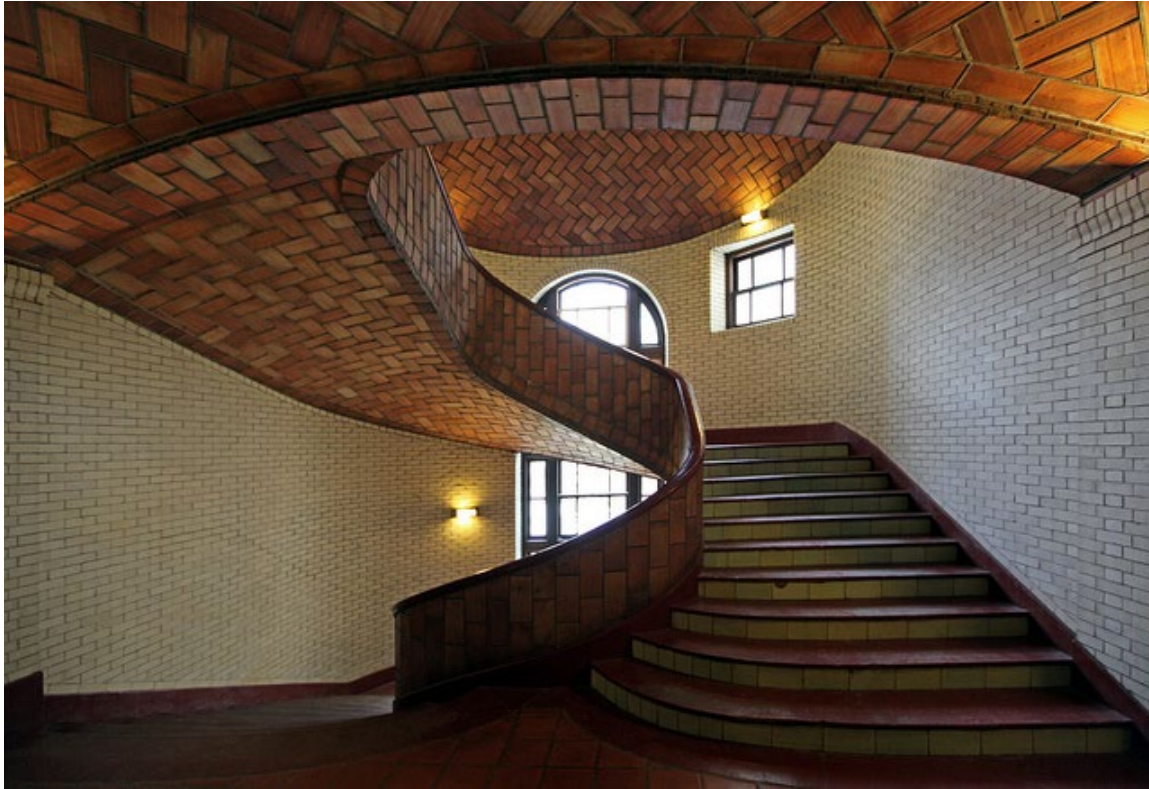
Guastavino stair in Baker Hall at CMU (Pittsburgh History and Landmarks Foundation)
