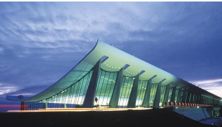
Dulles Main Terminal Expansion
